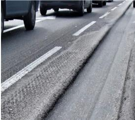
Fig.(1)Permanent deformation (Rutting)
